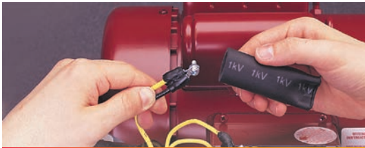
3M™ Pigtail Splicing
